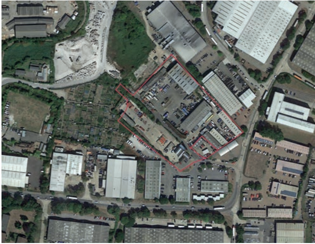
Site 95 & 102 aerial view
