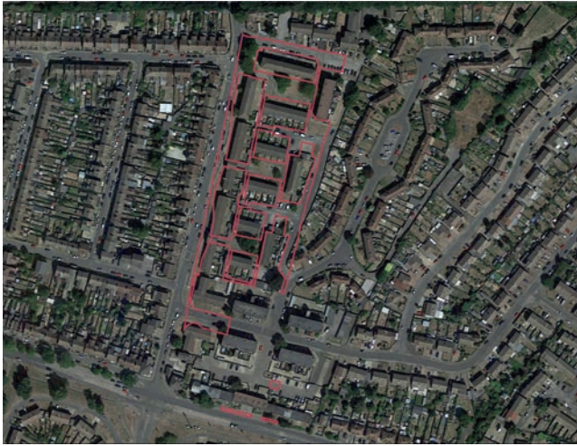
Site 140 aerial view
