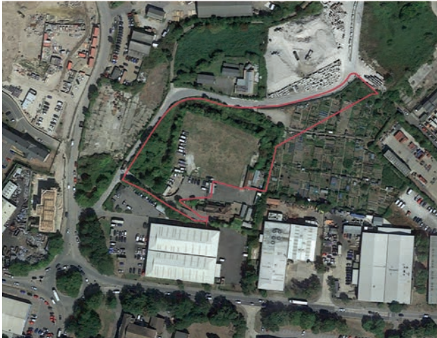
Site 106 aerial view
