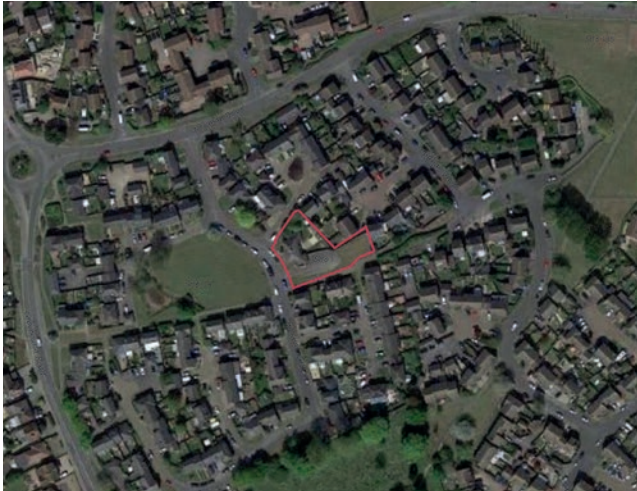
Site 1 aerial view
